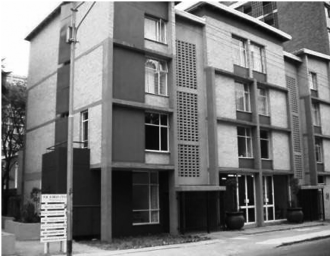
Figure 4.12 Jubilee Centre, Burgers Park Lane Source: Yeast City Housing (n.d.)
